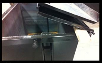
After marking both sides, use a block to hold the ez install lid up and out of the way for cutting the locking tab slots.
